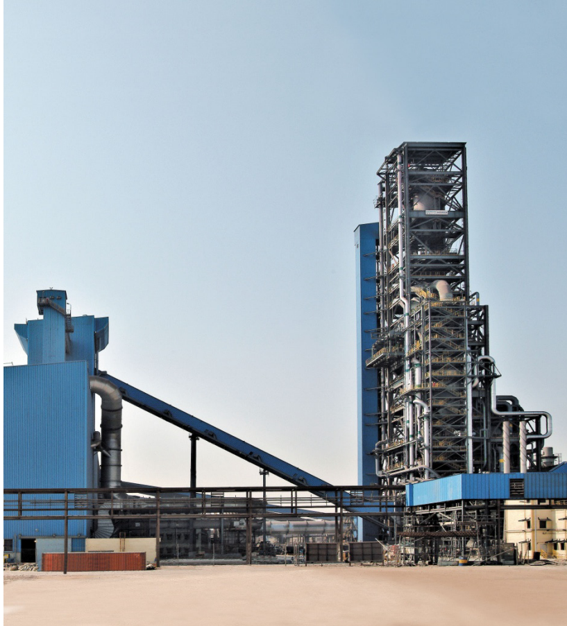
Figure 4 Hot Transport Conveyor at HADEED Module E
